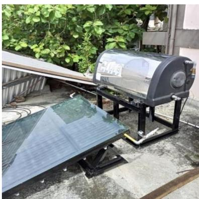
Gambar 2. Alat Solar Water Heater
